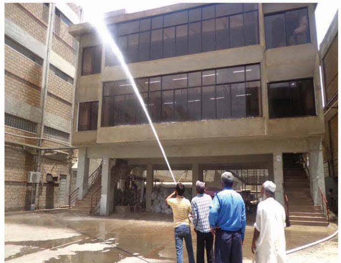
Fire hydrant drill training taking place at Unit 2
